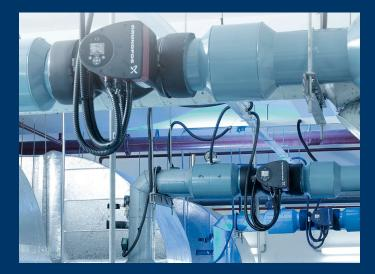
Installation was easy, with the initial pump configuration done using the Grundfos GO Remote app, and the adjustments to the flow limits were done directly in the BMS for each pump.
